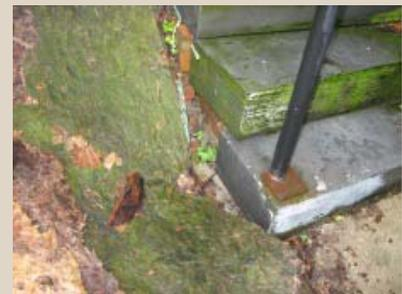
Cranmer House - Mold removal / basement cleaning through insurance co. Need to rebuild bilco door, stairs, seal coat problem area, and install commercial dehumidifier (optional: build porch roof over bilco door and steps). This cost needs to be paid by the Church. St. George's House - Electric in basement (completed.)
